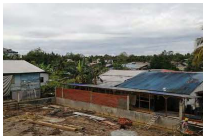
CSR - Rebuild wooden house for a family at neighbouring site
