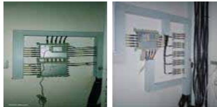
Satellite Master Antenna Television system
