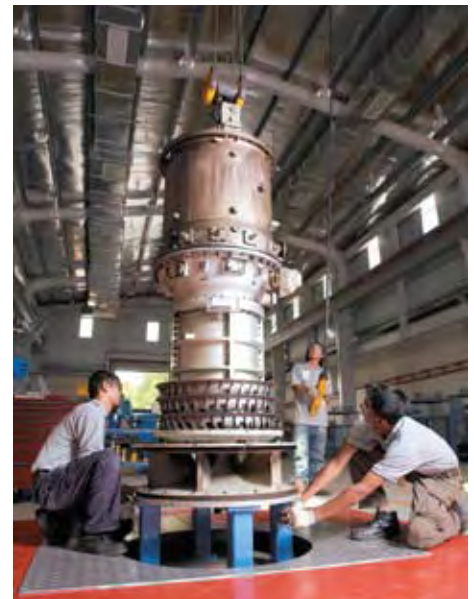
Gas Turbine assembly works
