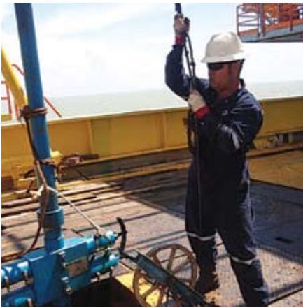
Installation of Pressure Control Lubricator
