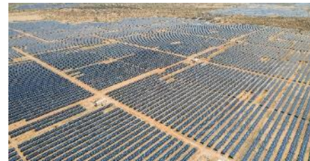
Bhadla Solar Park India
