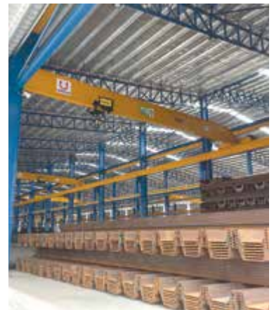
Electricity-powered overhead cranes
