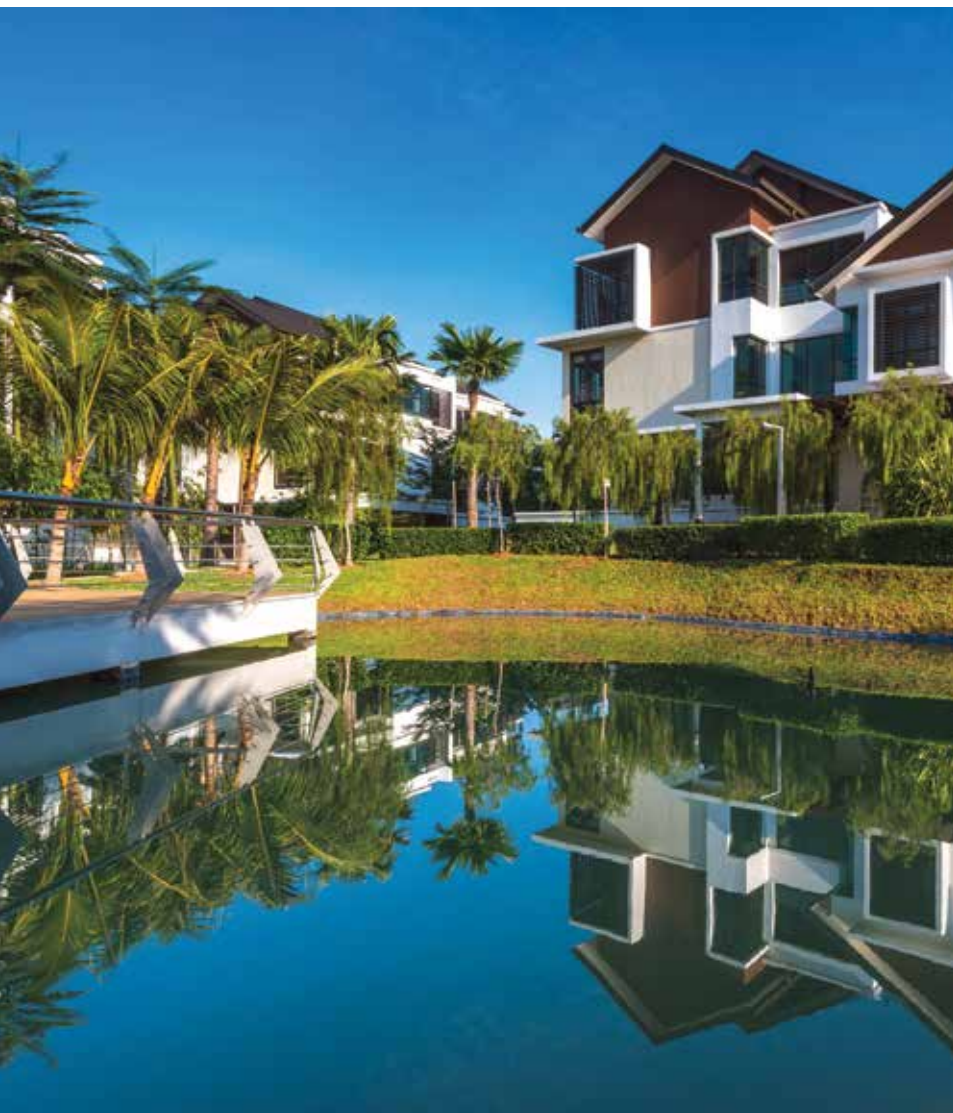
Rainwater Harvesting at Symphony Hills, Cyberjaya
