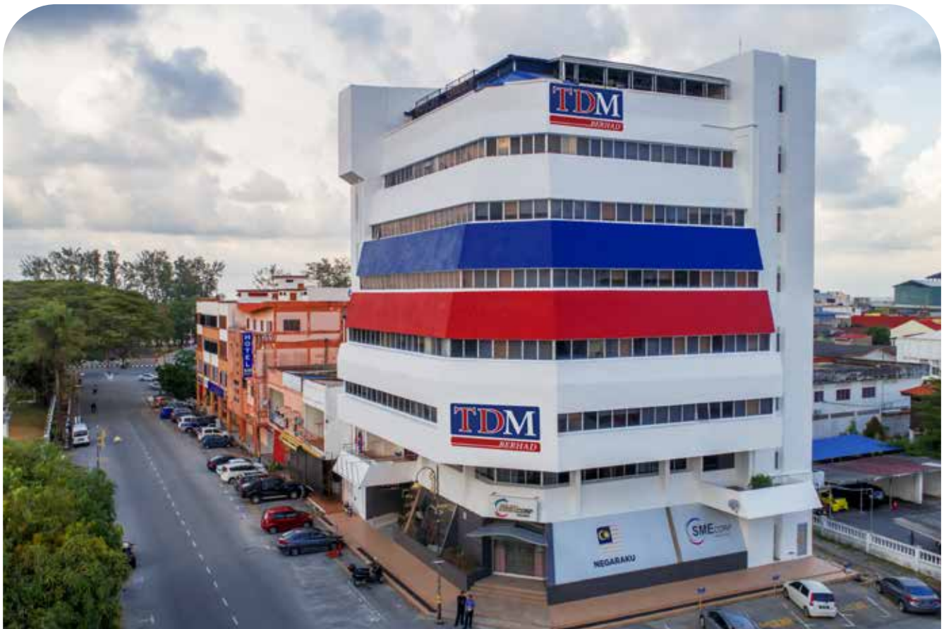
TDM Berhad's Headquarters in Kuala Terengganu.
