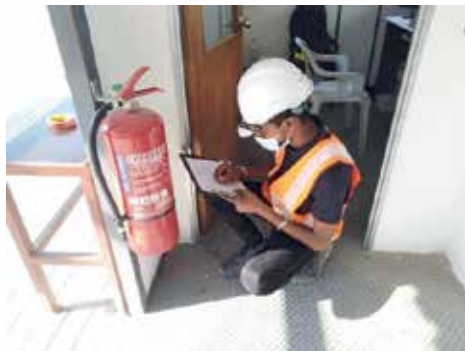
Inspection of Fire Extinguisher
