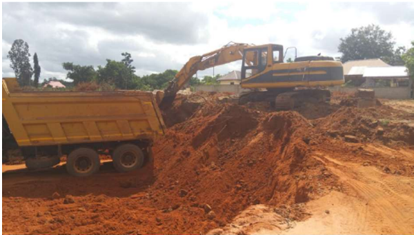
Backfilling in progress
