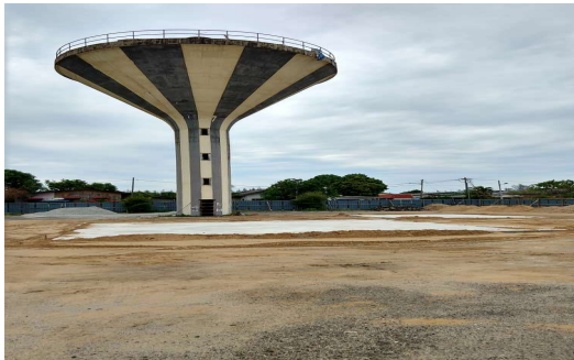
Telaga Daing- Slab for tank foundation
