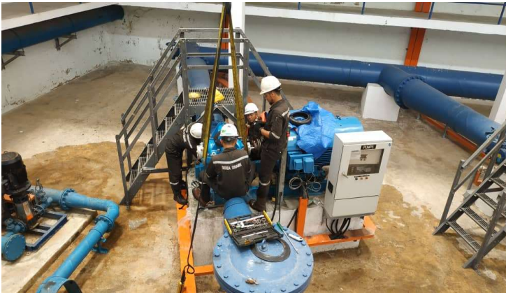
Kepong 2 WTP-(Retrofitting Works) Installation and alignment on Pump No 4 and Pump No 5
