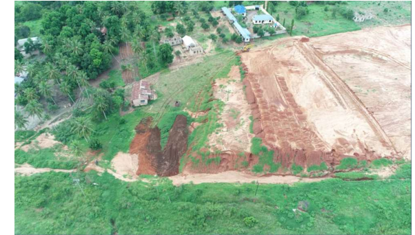
Excavation for silt trap
