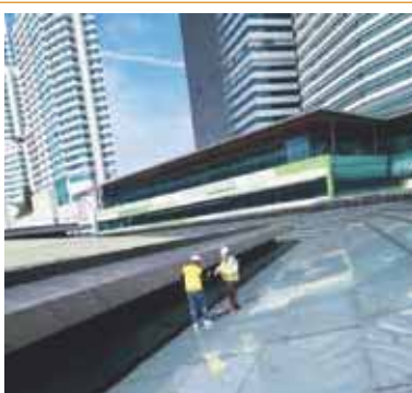
Figure 31: Upgrade of roof rainwater drainage system
