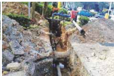
Figure 30: Replacement of underground domestic piping
