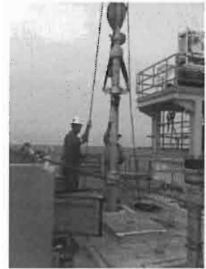
Lowering/raising slickline and wireline perforation tools
