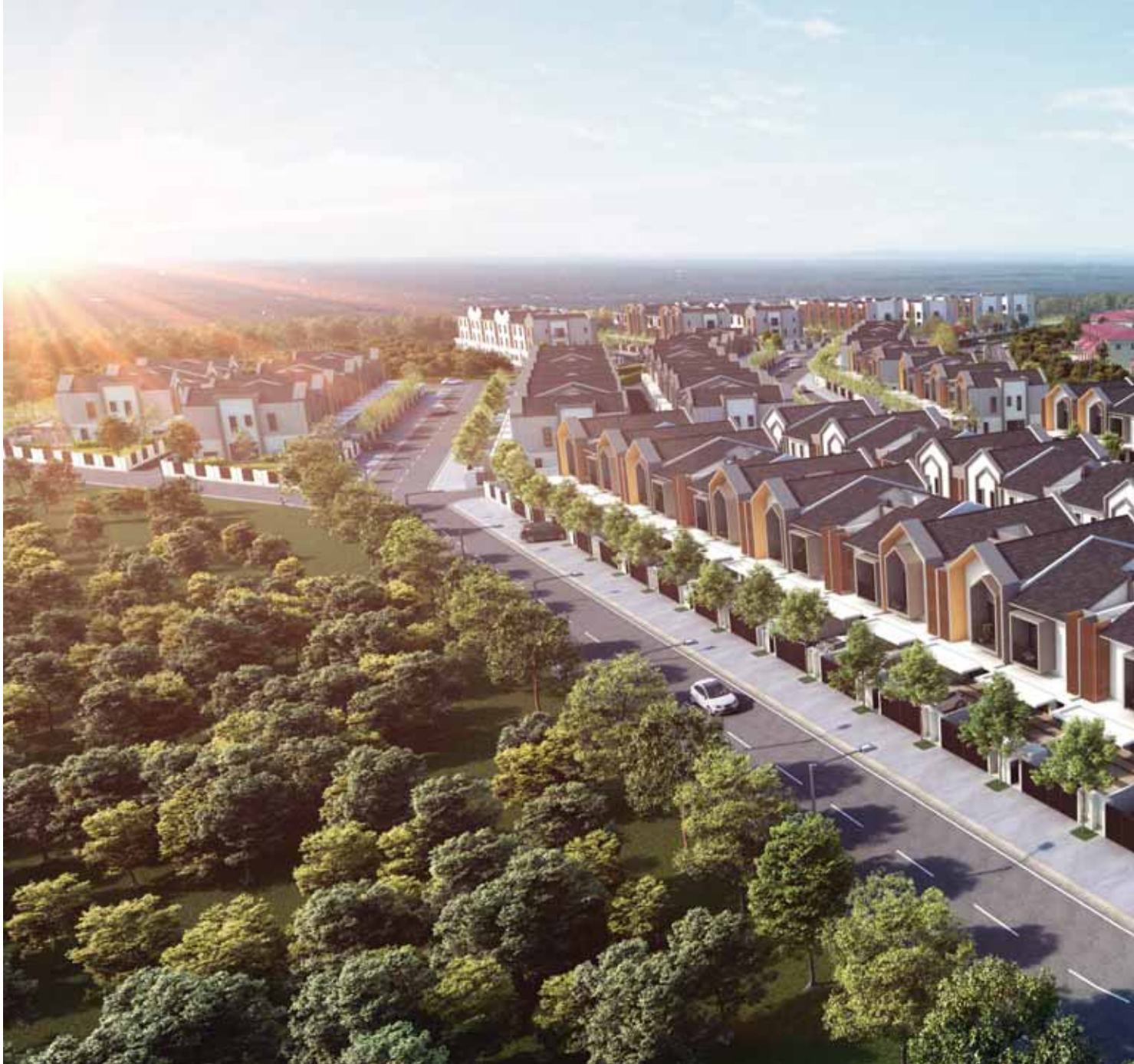
Aerial view of Diamond, Taman Putra Prima, Puchong
