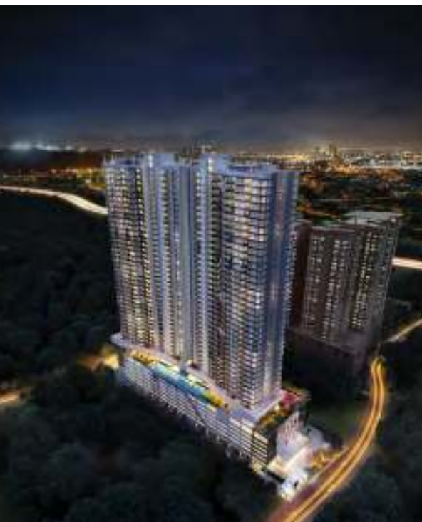
Artist's impression of high-rise development Inspirasi Mont'Kiara that was launched in February 2018
