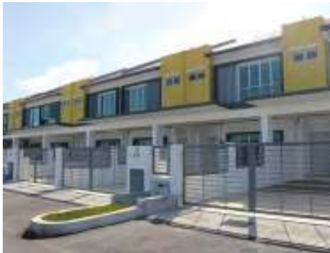
Completed units of double-storey terrace homes of Eugenia @ Hillpark 3 located in Semenyih
