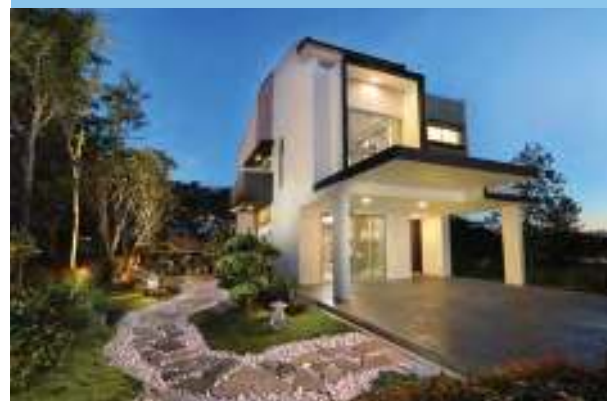
Show unit of Kajang 2 Precinct 2 Phase 3 (Midori) and 4 (Hiroki) double-storey terrace was completed for customer viewing during the launching ceremony in November 2017
