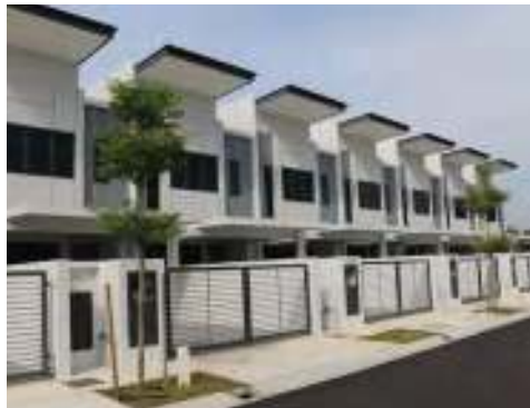
Completed units of double-storey terrace homes of Kajang East Precinct 4 located in Semenyih
