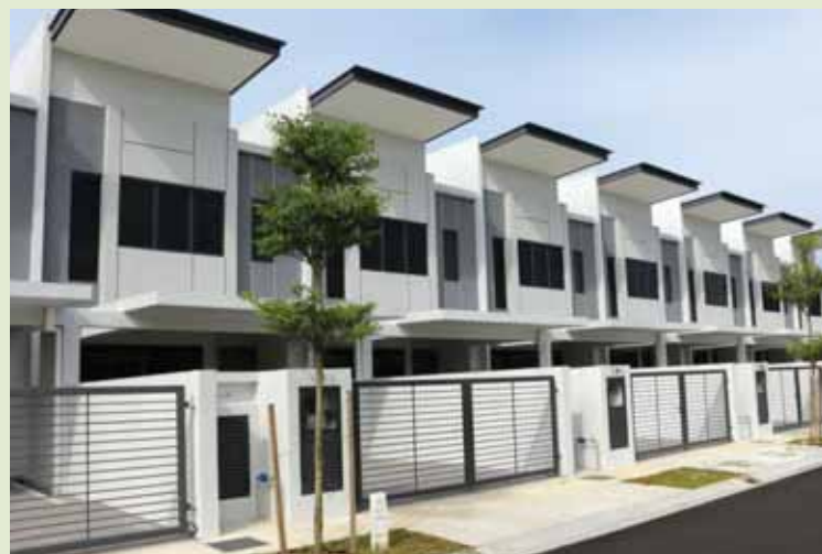
Kajang East Precinct 4 achieved QCLASSIC scoring of 83% in April 2017
