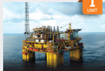
SEMI-SUBMERSIBLE FLOATING PRODUCTION SYSTEM (SEMI-FPS)
