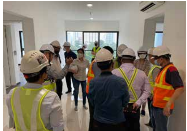
Performing routine site inspections and on-site training to monitor the quality of craftsmanship throughout the construction progress.
