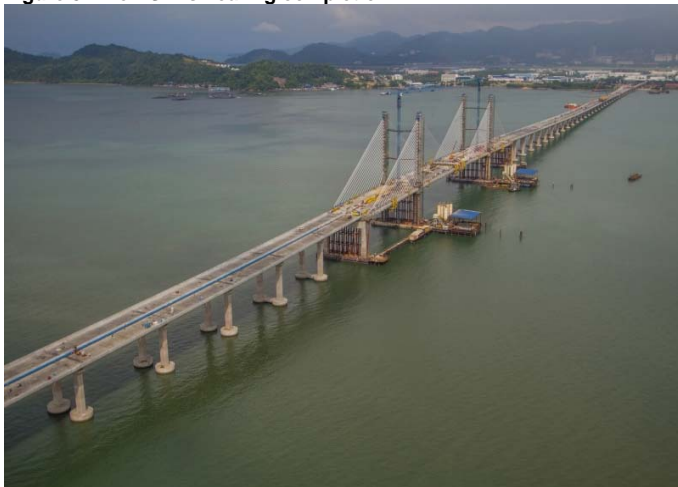
Figure 5 The PSB is nearing completion
