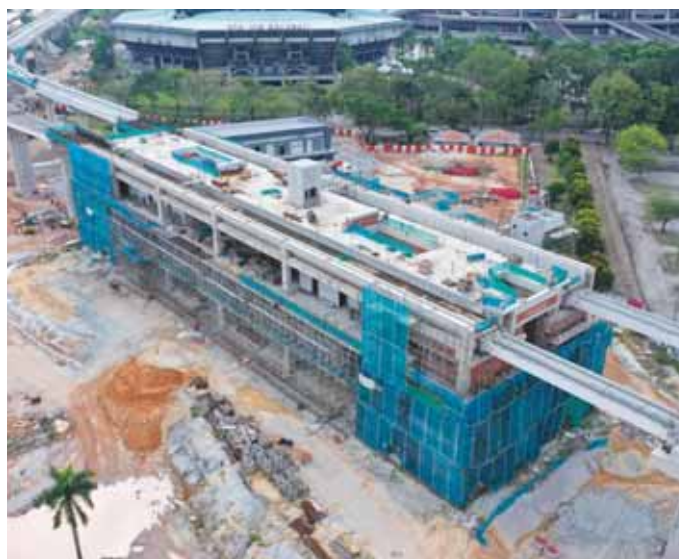
LRT3 (GS04) - Stadium Station, Shah Alam
