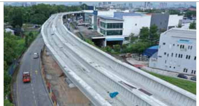
Viaduct works in progress and cast in situ extended pier cap
