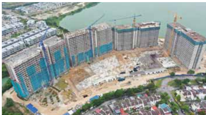
E'Island Lake Haven - Overall Site View
