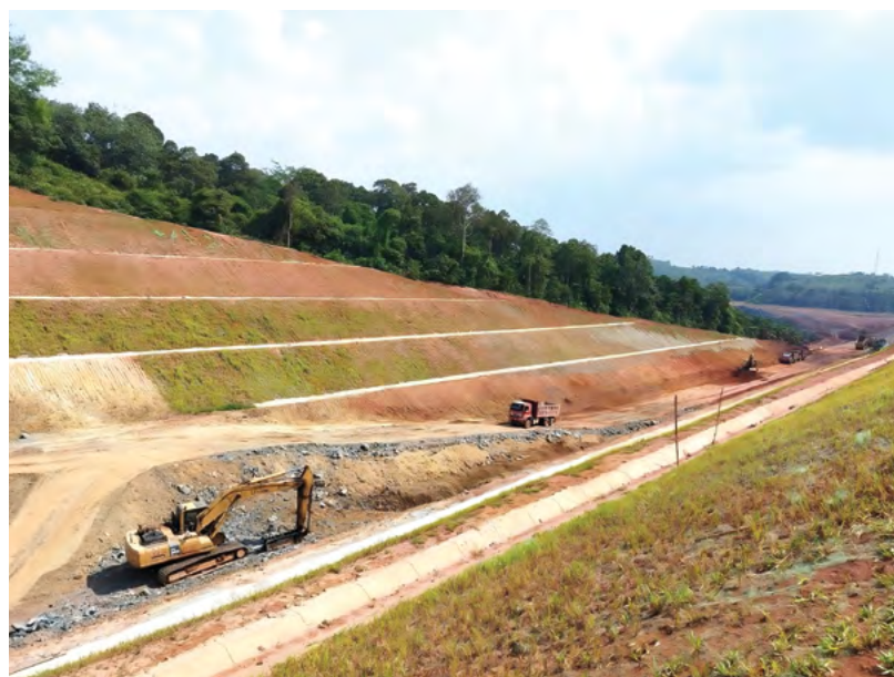
ECRL Section 6 (CH409+250 to CH409+570): Removal of soil and rock
