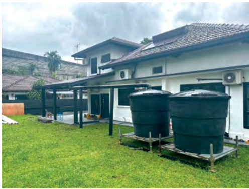
Rainwater harvesting system installed at RTS Link
