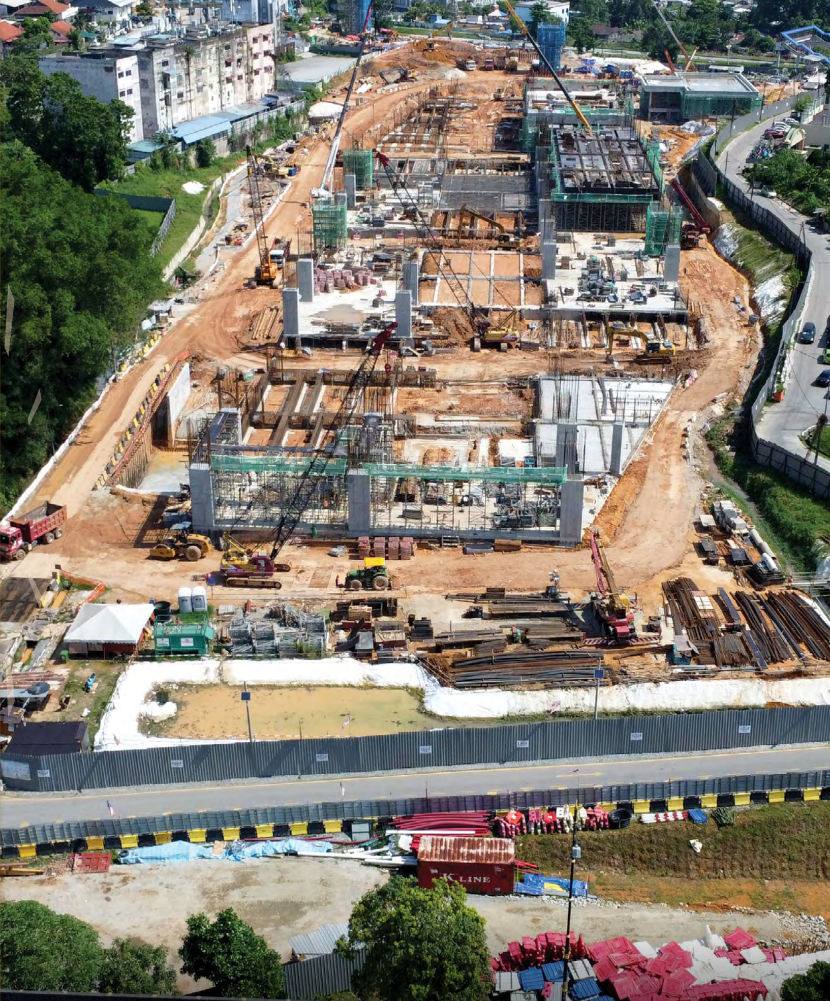
RTS Package 6 - Aerial view of Depot construction
