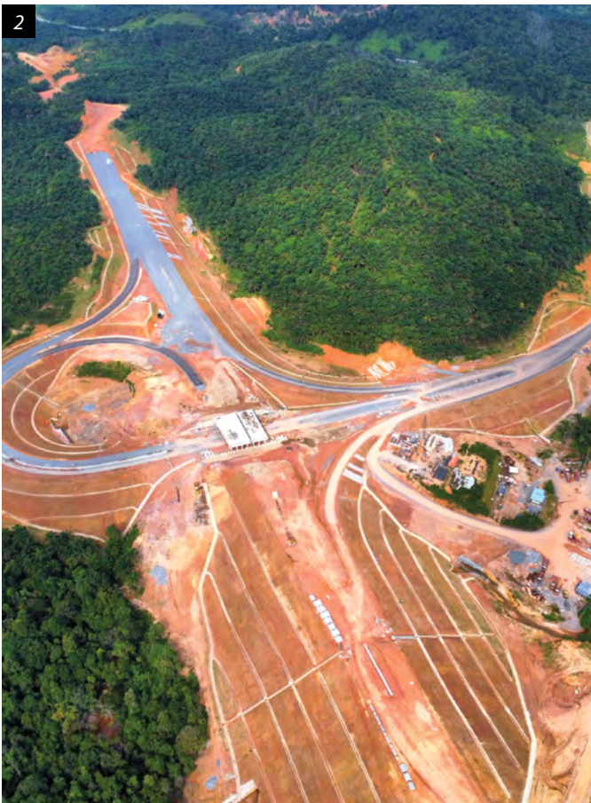
2. Construction of Interchange for Central Spine Road, Section 2B
