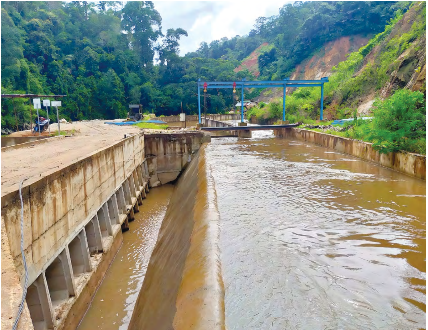
Vicinity view on Mini-hydro Power Plant Spillway
