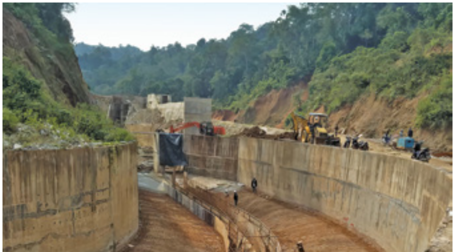
▲ Mini-hydro Power Plant waterway
