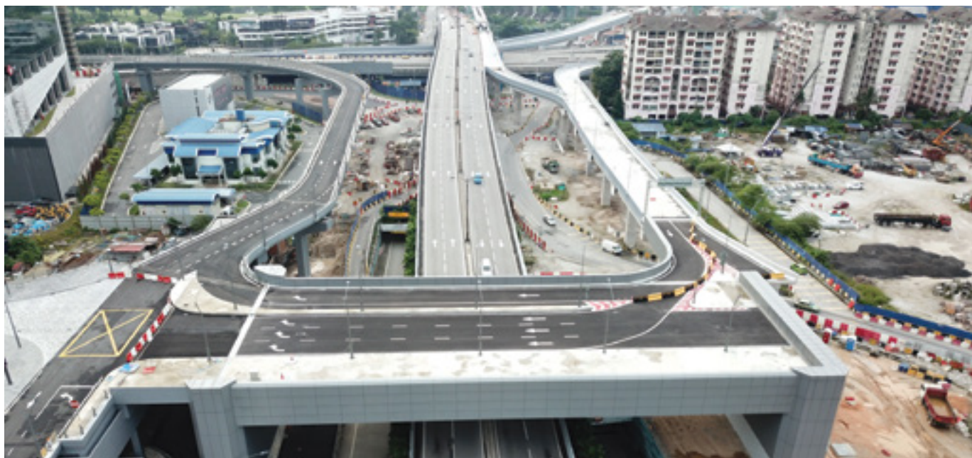
▲ North-South Steel Bridge at Tun Razak Exchange
