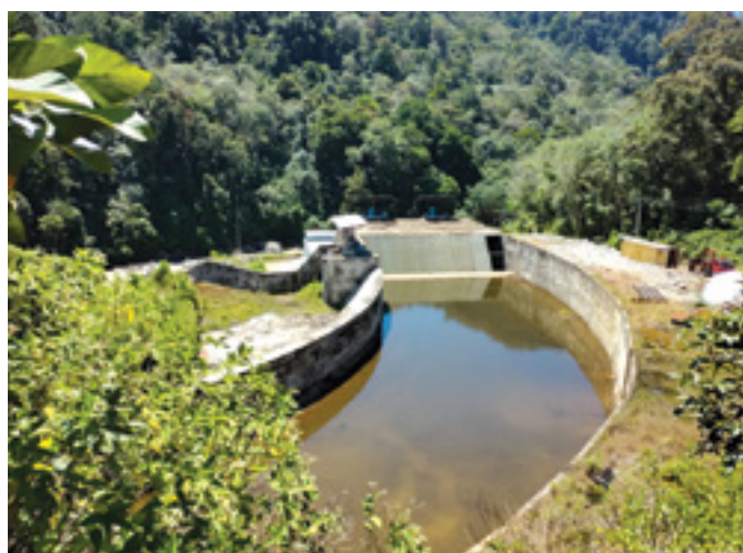
▲ Vicinity view on Headpond, 9MW Mini-hydro Power Plant
