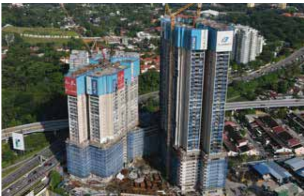
Drone image taken at Duta Park project
