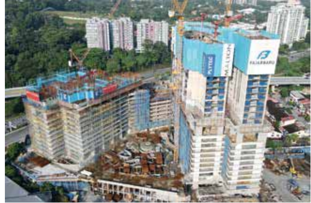
Construction of Duta Park Residences
