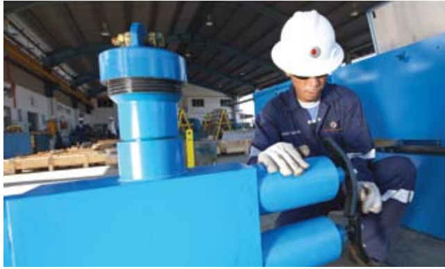
Assembling of BOP prior to pressure testing
