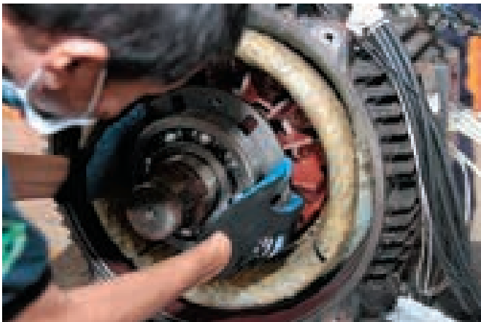
Overhauling of motor
