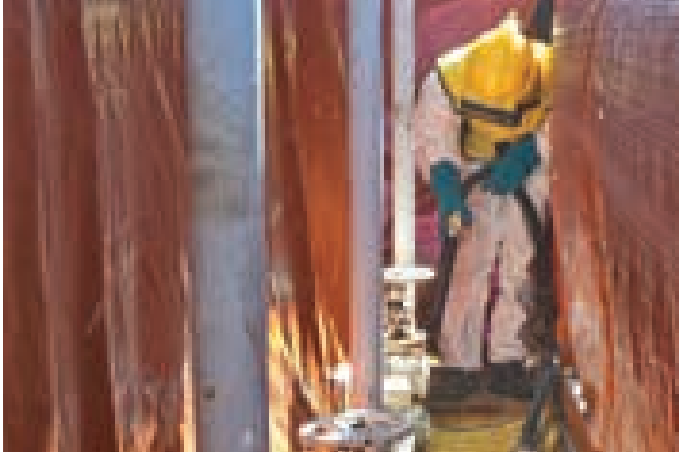
Blasting using Sponge Jet technology
