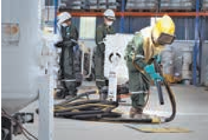
Blasting using Sponge Jet Technology
