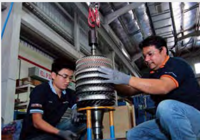
Installation of compressor rotor stators and spacer rings
