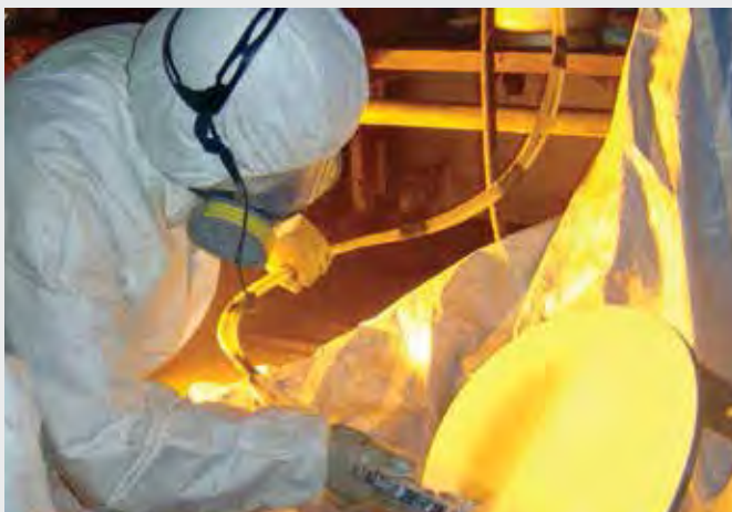
Internal lining coating
