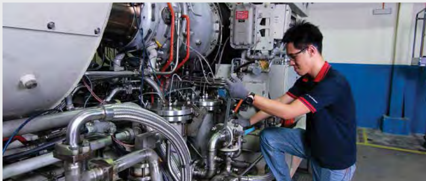
Installation of lube oil connections
