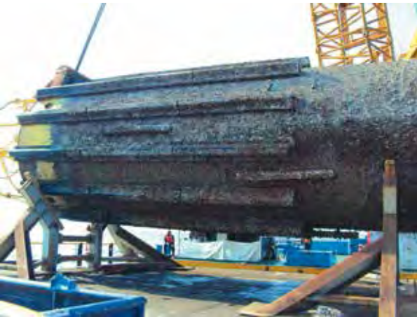
Aggressive Coating Removal
