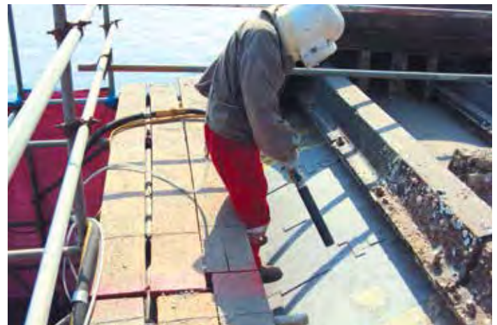
Sponge-Jet Abrasive Blasting
