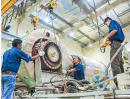
Overhauling Gas Turbine
