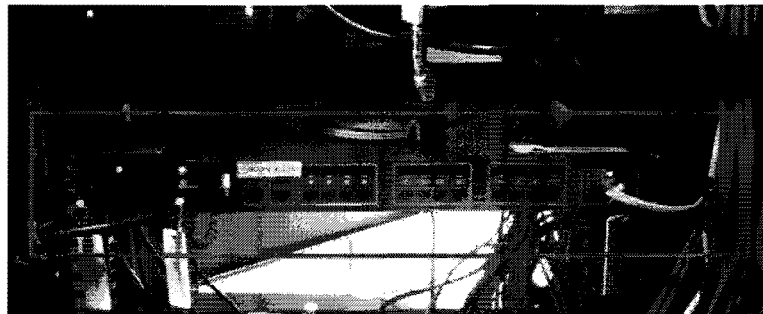
Network equipment that we installed for our customer
