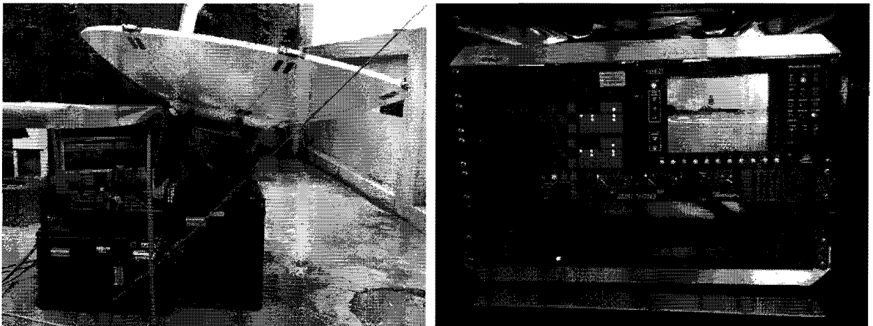
Our flyaway VSAT ground station dish (left) and network equipment (right)
