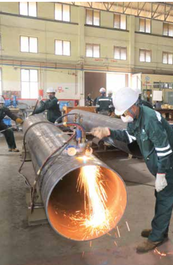
Fabrication works of a Floating, Production, Storage & Offloading (FPSO) project sea water cooling pipes undertaken at BNS
