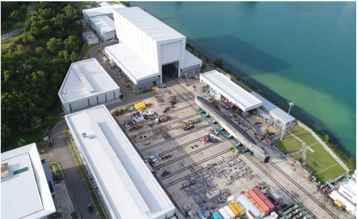
Aerial view of the RMN Yard in Sepang Bay, Kota Kinabalu operated and managed by BDNC, our JV company with France's Naval Group. BDNC, supported by our wholly owned subsidiary BHIC Submarine Engineering Services Sdn Bhd, is entrusted by RMN to provide In-Service Support and carry out Refit works for RMN's fleet of Scorpene submarines
