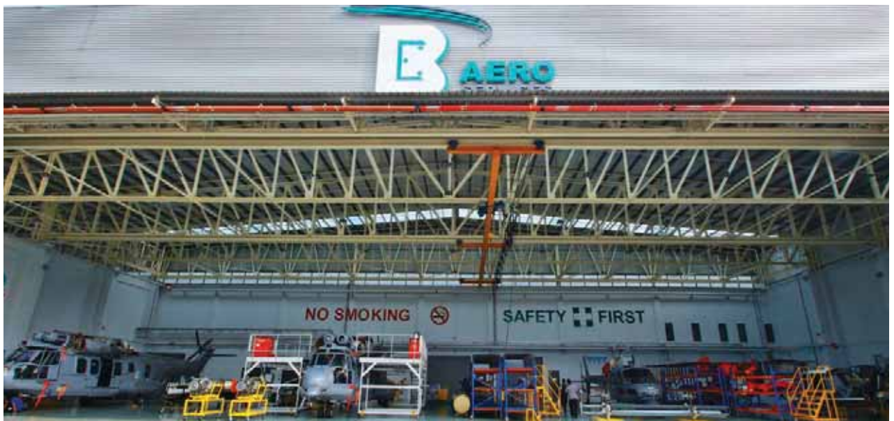
BHICAS is capable of undertaking a maximum of four helicopter repair works at a time
