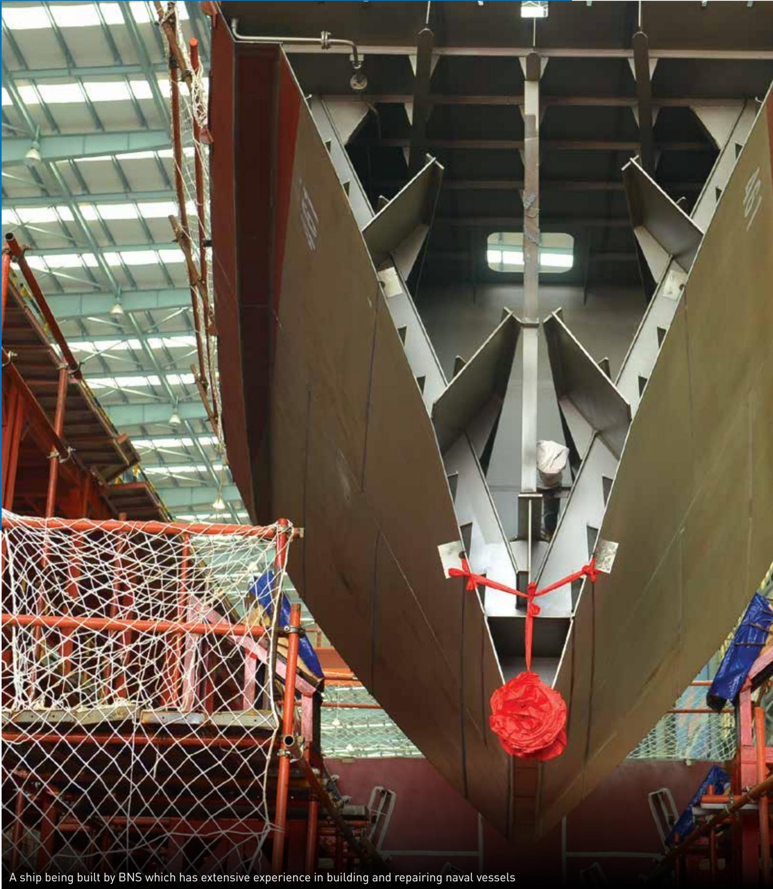
A ship being built by BNS which has extensive experience in building and repairing naval vessels
