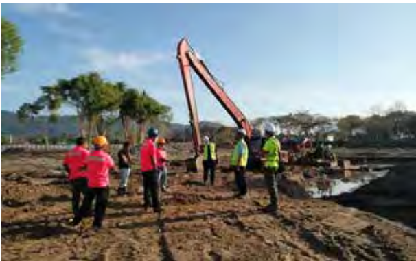
01 ESH Visit & Site Safety Evaluation at Sand Management LPO Project
