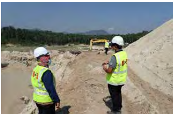
02 ESH Site Inspection at Sand Management Quarry Sungai Ular, Kulim
