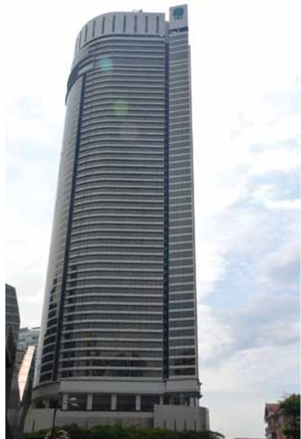
Banyan Tree KL (Engineering Division).
