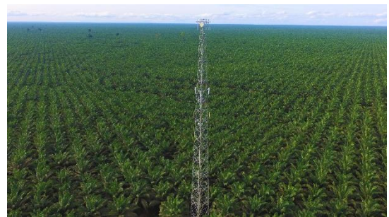
Mobile telecommunications tower
