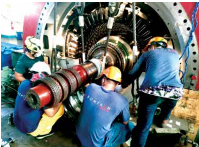
Major Overhauling of Generator
