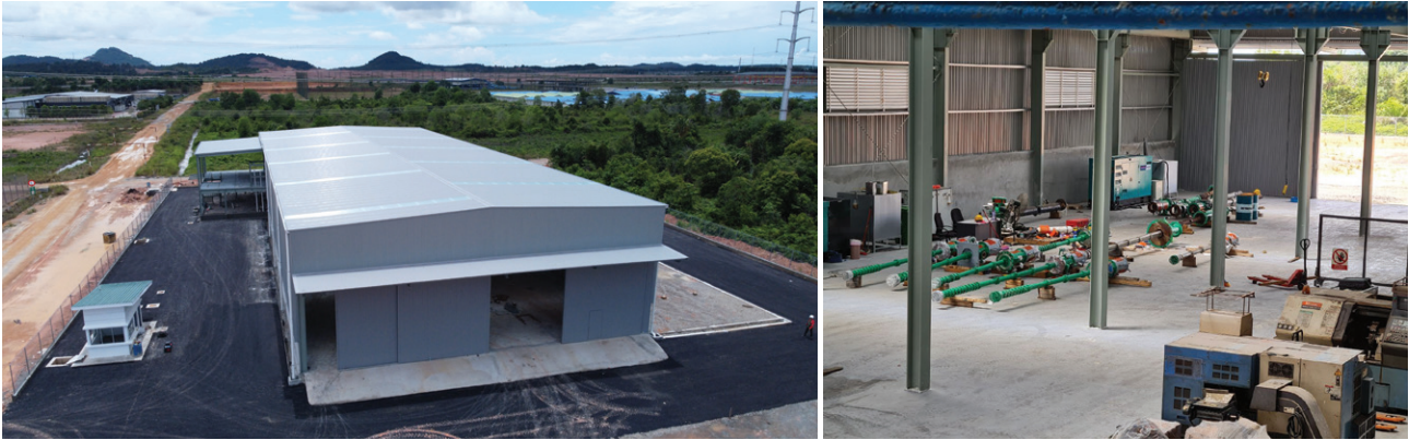
Aerial view of our New Workshop at Pengerang, Johor in December 2021
