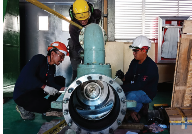
Hydraulic Installation Works
