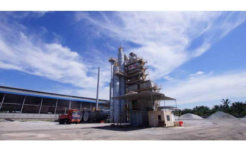
The plant is being equipped with a batching system with the capability of producing 40,000 tonnes of asphaltic bituminous mix products monthly. KKPP is the largest addition to BDB Infra's production and manufacturing facilities.
