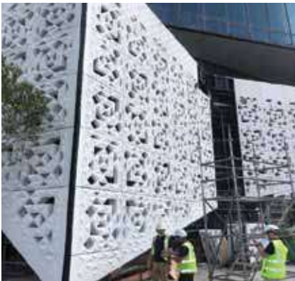
Picture: Bukit Jalil Pavilion 2 Shopping Mall – Façade walls constructed using UHPC that are highly customised, curved with three pattern features, pre-finish with everlasting pigmented homogeneous colours. Large and lightweight panels allow quick, fast track construction.
