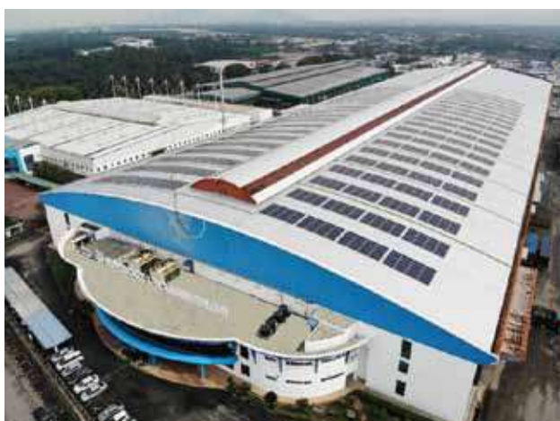
Picture: 998 kilowatts peak (kWp) Solar PV system installed by Solarvest at GS Paperboard and Packaging Sdn Bhd's rooftop located at Sungai Bakap, Penang. The company will offset up to 953 tonnes of CO 2 which is equivalent to planting 28,440 of trees.
