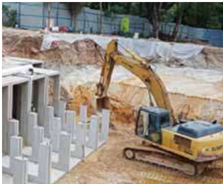
Picture: Lifting of G-Cast Eco-Modules (customised underground stormwater storage tanking system) for installation to On-Site Detention Project located at Taman Botani Kuala Lumpur own by DBKL.
