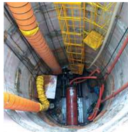
Picture: Polymer concrete pipe with stainless steel jacket was designed by MI Polymer Concrete Pipes Sdn Bhd, tested, supplied and installed at PUB’s Project
