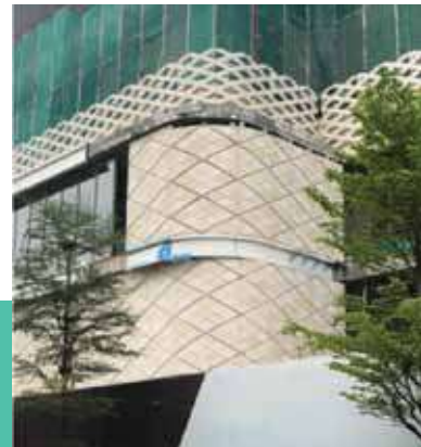
Picture: HSBC Bank Malaysia Berhad's new RM1 billion headquarter is located at the Tun Razak Exchange main entrance facade features constructed with G-Cast UHPC's panel (design and build project)
