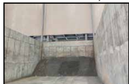
Coal Bottom Ash Storage (Sheltered Stockpile)
