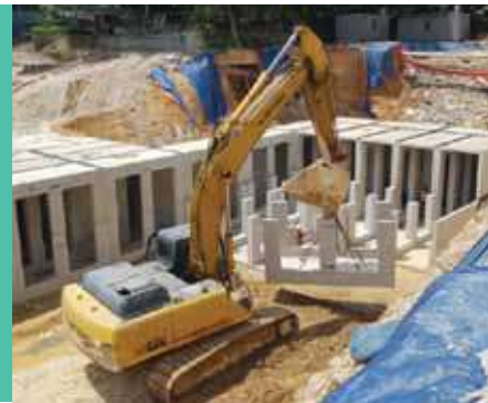
Picture: Lifting of G-Cast Eco-Modules (customised underground stormwater storage tanking system) for installation to On-Site Detention Project located at Taman Botani Kuala Lumpur own by DBKL.
