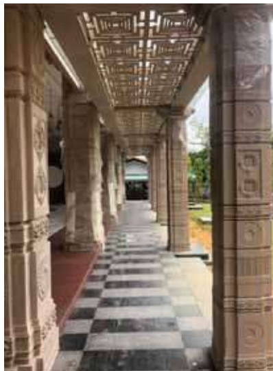
Picture: Shree Lakshmi Narayan Temple located at Jalan Kasipillay, Kampung Kasipillay, Kuala Lumpur – Temple dome tower structure construction using UHPC with high detailing finishing and design
