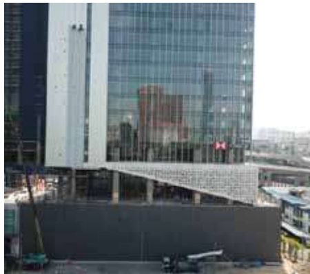
Picture: HSBC Bank Malaysia Berhad's new RM1 billion headquarter is located at the Tun Razak Exchange main entrance facade features constructed with G-Cast UHPC's panel (design and build project)
