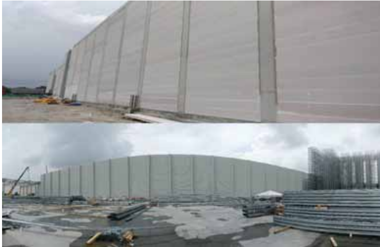
Picture: Starken AAC supplies the AAC panels to Ikea Distribution Center at Pulau Indah, Klang. The AAC panels are used as the wall panels for the Center.
