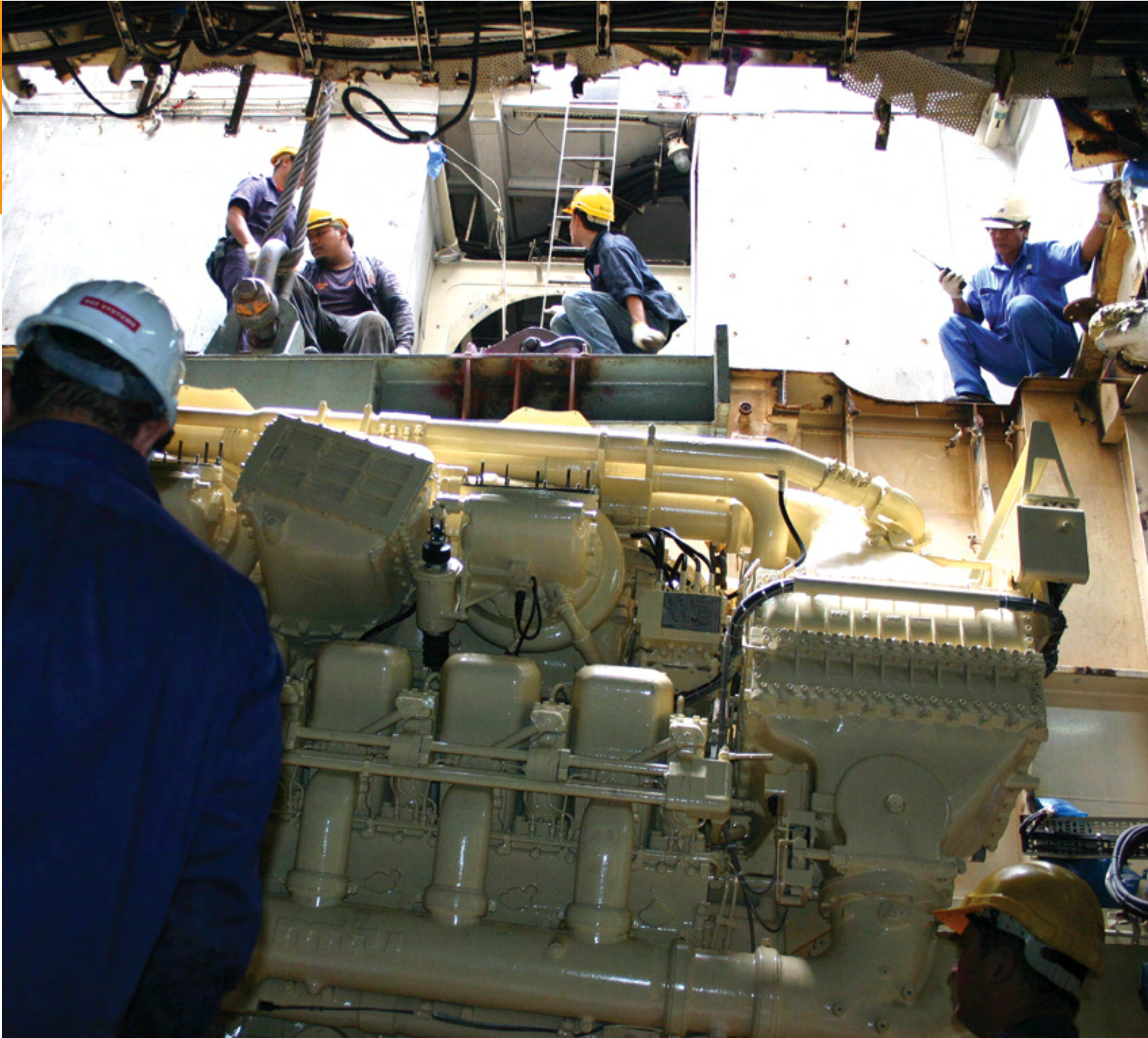
Engine installation for Navy vessel at Lumut Yard.
