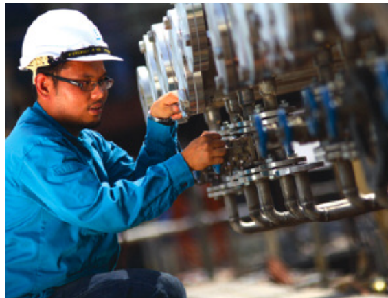
Technical personnel monitoring piping installation.
