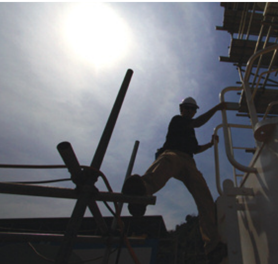
Work in progress at tanker, Jerejak Yard.
