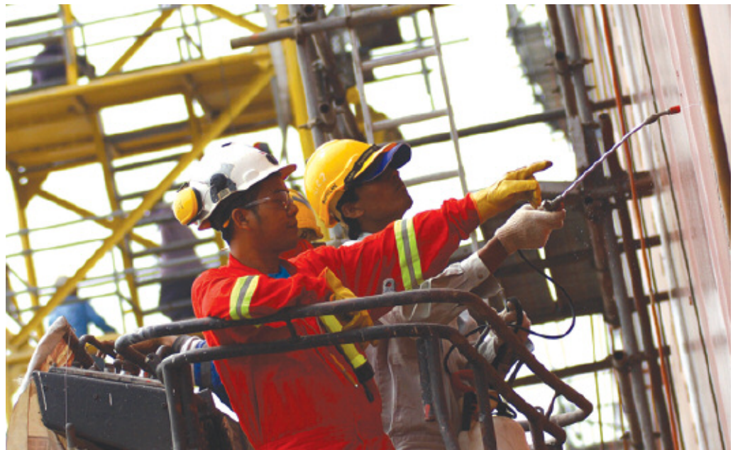
Thorough tank air test conducted to ensure quality at Jerejak Yard.
